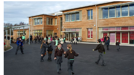
Oak Meadow Primary School Passivhaus (Source: Architype)
